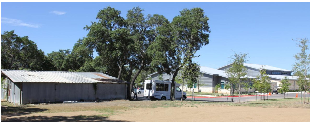
Pictured above is the old pantry to the left and the new facility to the right
